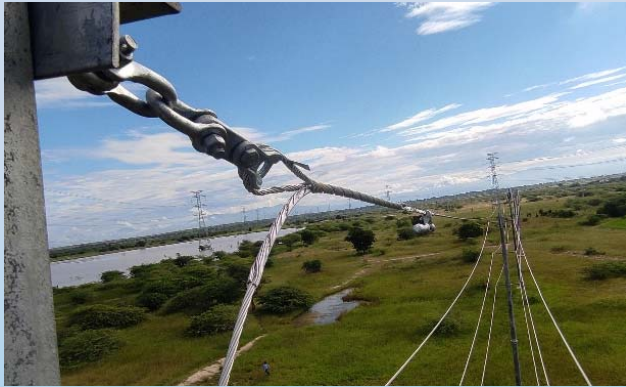
OPGW Cable combines the functions of grounding and communications
