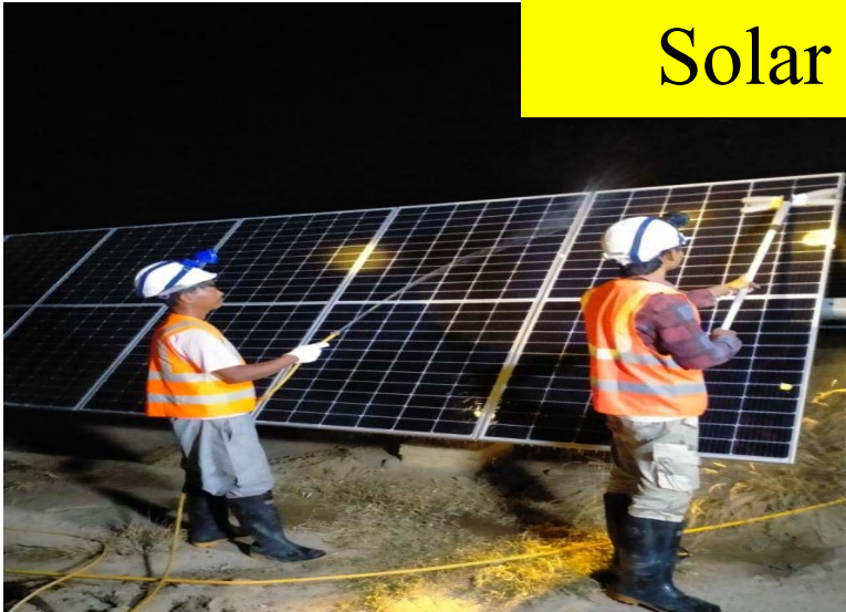
PV Modules Cleaning
